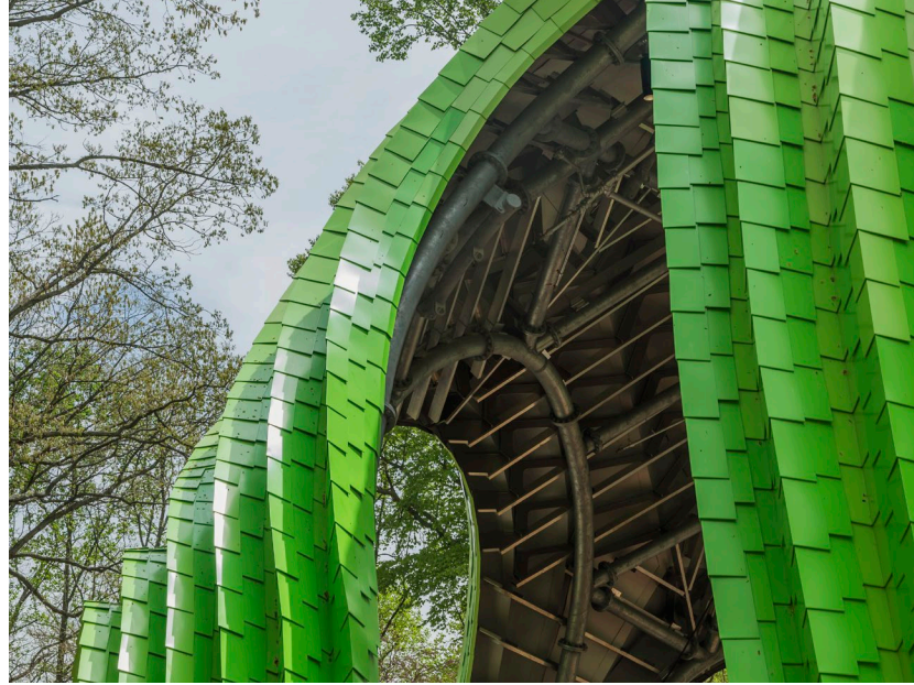
Chrysalis as-built: close-up views of aluminum shingled skins.
