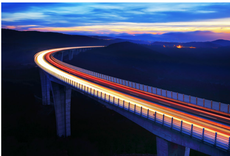
With VDC: Connections between construction processes are seamless.
