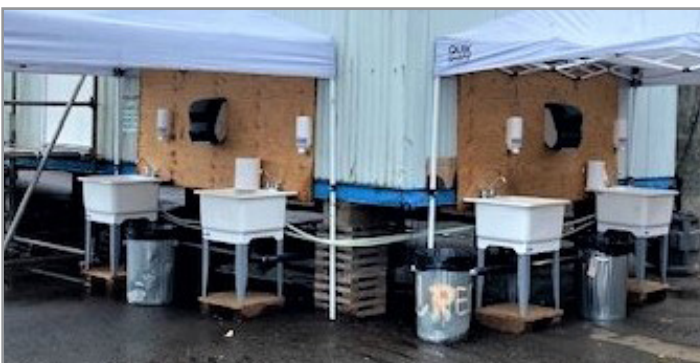
Hand-wash facilities 6 feet apart. (Photo courtesy of Boilermakers – CIMS Ltd.)
