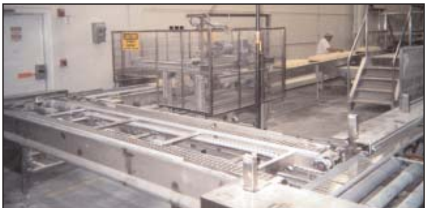
All machine guards and handrails were fabricated by TAL-MAR.
