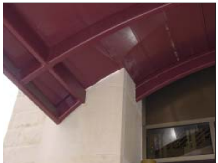
An angle support should be under the panels.
