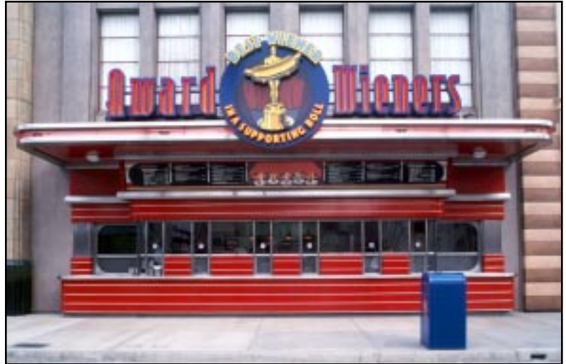
The exterior panels of Award Wieners are powder-coated red aluminum. This project has no exposed fasteners.
