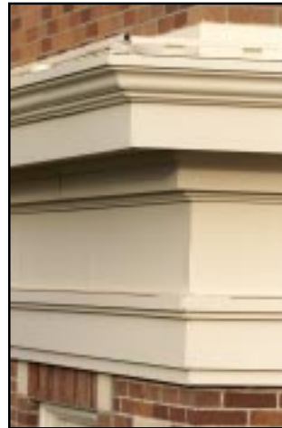
Far Left: Monroe Hall now features renovated cornices that preserve its historical facade.
