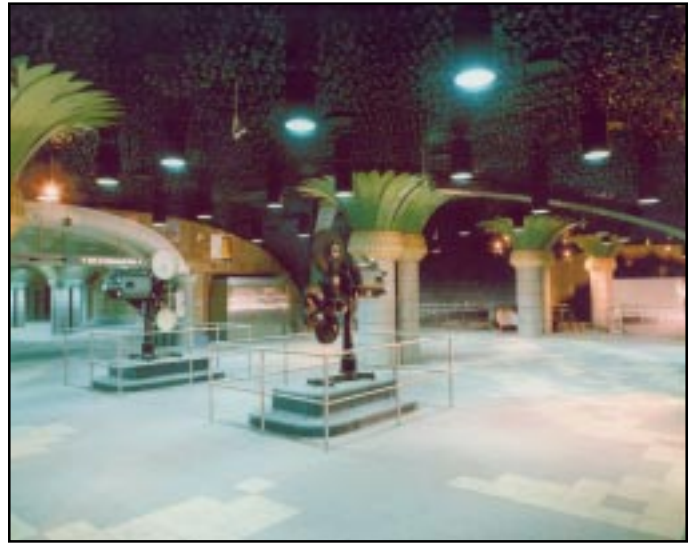
The Hollywood/Vine station features decorative palm leaves laser cut from .125-inch aluminum plate and powder coated.
