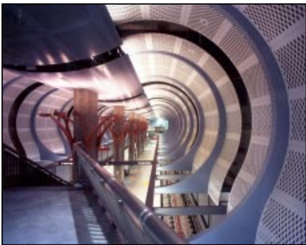
The North Hollywood station's hypnotic circular pattern was achieved with .090-inch aluminum panels placed in a radius pattern with a graduating perforations.
