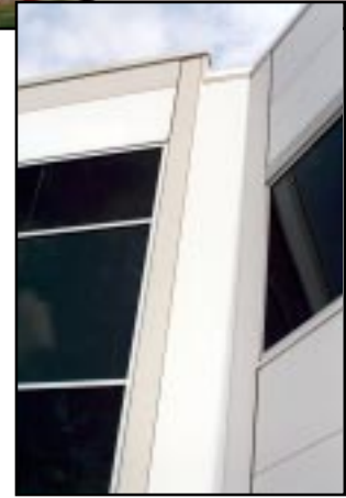
View of the panels and the aluminum color bands that give the building a decorative detail.
