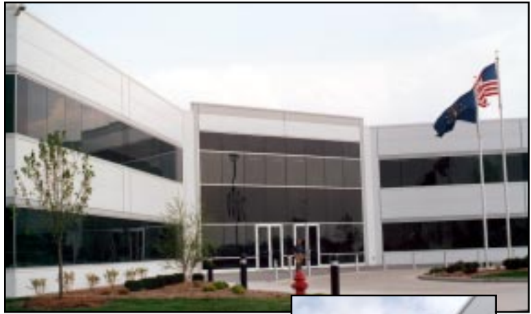
The exterior view of the Guide corporate headquarters features the clean crisp lines of the Metl-Span panels.
