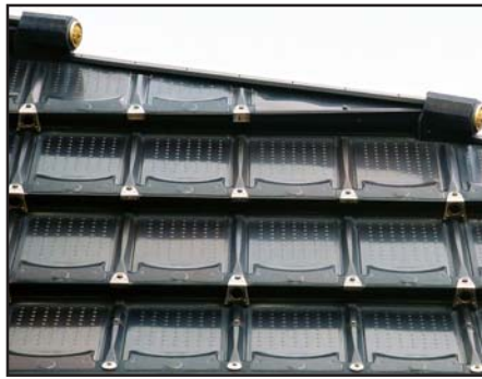
Figure 1: Shakaden Temple roof. Photo courtesy of the Nickel Institute
