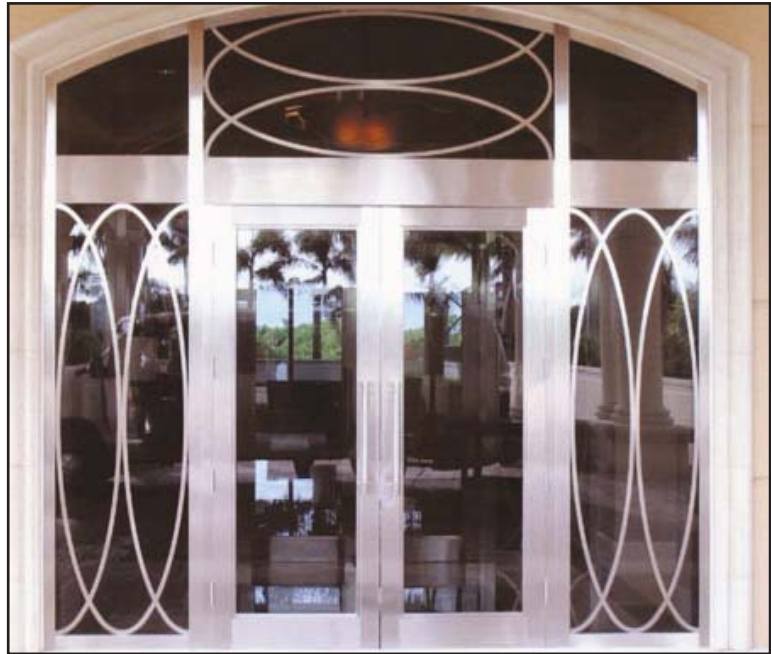
SMACNA contractor MetalFab Inc. of San Antonio, Fla., clad the existing entrance of this Bonita Springs condominium with stainless steel and applied laser cut pieces to the windows.
