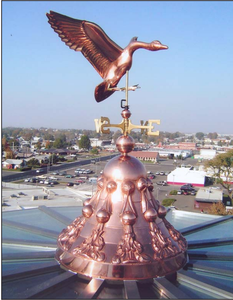
The very top of the dome was handmade.
