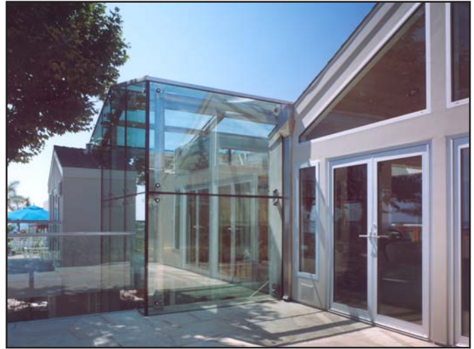
The custom home remodel included a glass elevator enclosure structure, sheet metal crickets with coping, leader head and stainless steel downspout.
