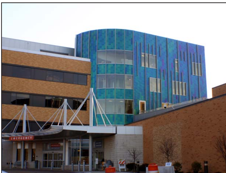
The $1,055,000 job included stainless steel metal flat seam wall panels or metal shingles.
