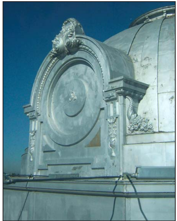
The existing dome which was galvanized with zinc ornamentation.
