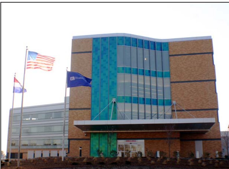
The Rimex green stainless steel material was challenging to work with due to its green anodized finish that could not be repaired, if scratched.
