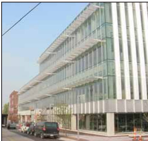
The $1,020,000 job included the fabrication and installation of 104,696 pounds of aluminum as well as 53,082 square feet of post clear anodized aluminum.
