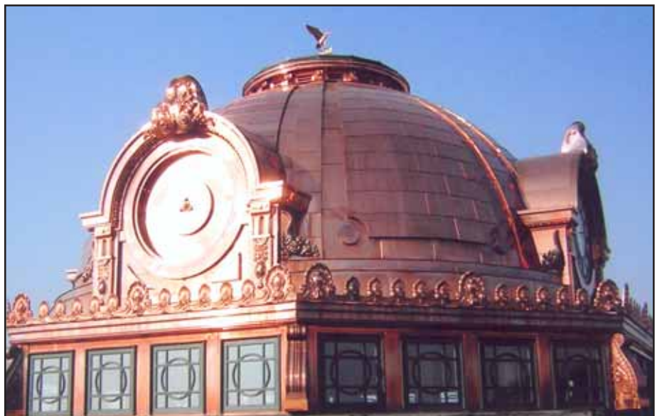
Completed Restoration of the Franklin County Courthouse.
