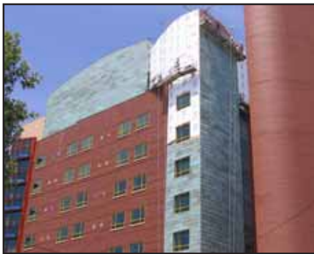
Installation was achieved using aerial lifts and suspended scaffolding.
