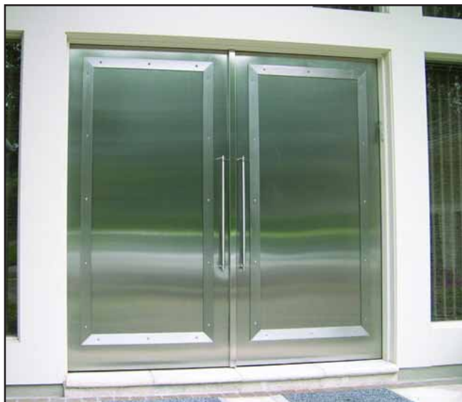
A 16 gage #3 stainless steel sheet was used to clad over the existing doors with a 38 inch by 3 inch stainless steel brush finished flat bar.
