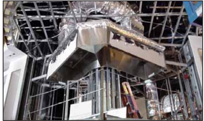
A 304 stainless steel with a #4 finish was used for all of the food service equipment.
