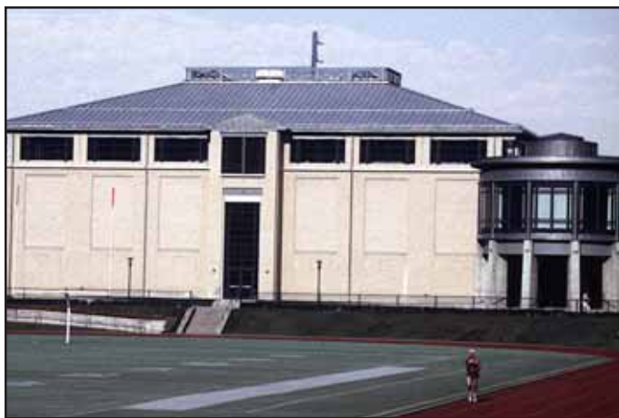
Figure 2: Terne-coated stainless steel roof and elevated wall panels on the Carnegie Mellon University student union building, Photo courtesy of Nickel Institute, Catherine Houska photographer.
