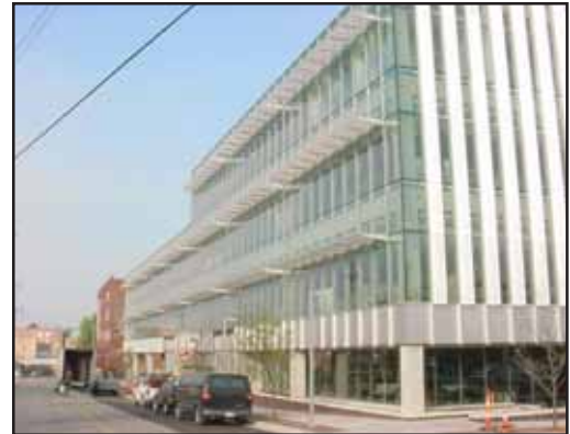
Left: FCM Custom Metals' work on the project included wall panels, vertical perforated sunshades, horizontal sunshades and interior light shelves.
