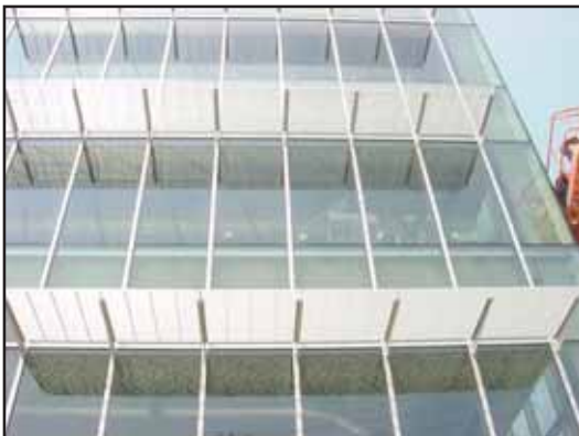
Left: FCM Custom Metals' work on the project included wall panels, vertical perforated sunshades, horizontal sunshades and interior light shelves.
