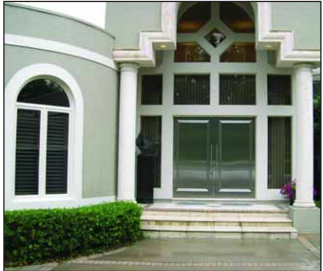
Overall this design build project required approximately 60 man-hours for the fabrication and installation of the doors.
