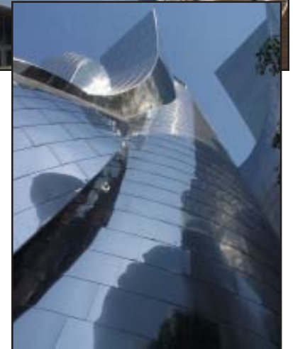
The strict guidelines of Frank Gehry's design did not allow for any defects in the bright annealed, Type 316, 24-gage stainless steel panels.
