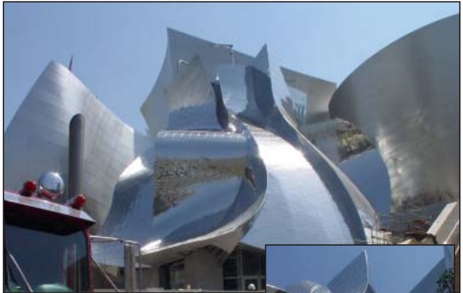
Occupying a city block in downtown Los Angeles, the striking mirrored exterior of the Disney Concert Hall reflects its famous neighborhood – just south of the Dorothy Chandler Pavilion, home of the Academy Awards.
