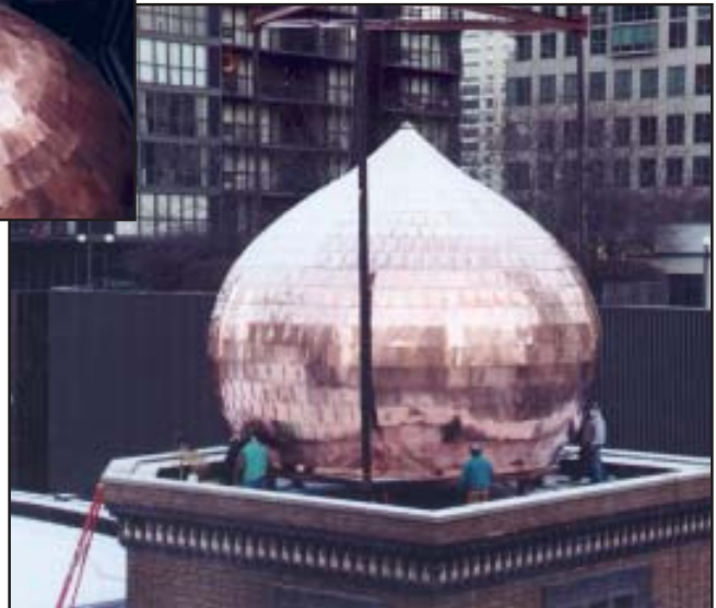
Measuring 28 feet at the widest point, the copper onion domes were placed by crane back in their original positions. With more than 1,550 copper sheets on each dome, craftsmen cut every panel to exact measurements for each course around the dome.
