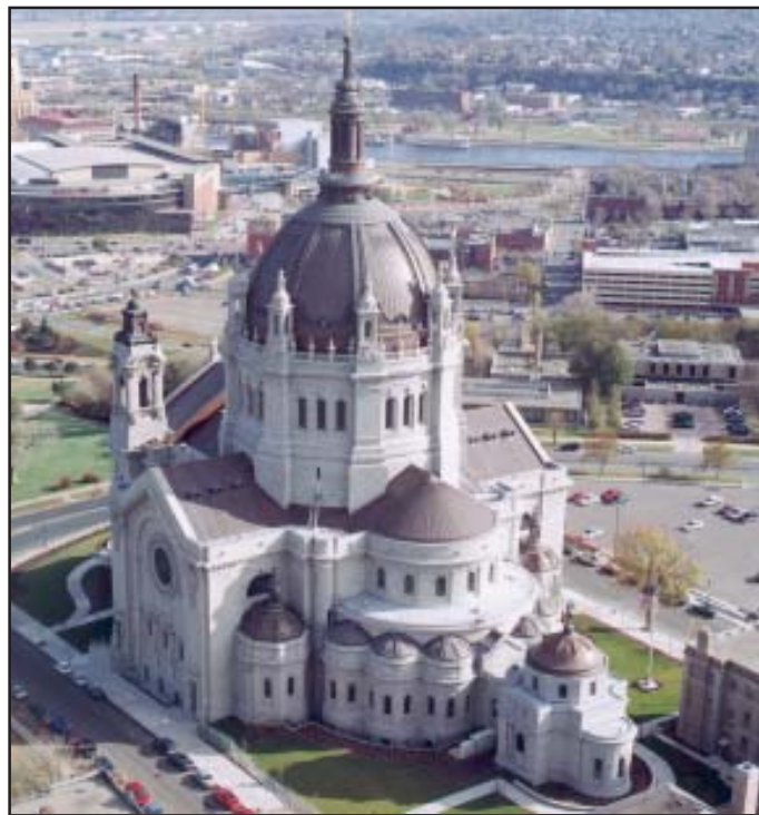
The complete $30 million restoration and renovation of the Cathedral of Saint Paul included roof replacement, copper restoration, exterior granite repair, interior building repairs, electrical system renovations and mechanical system renovations.
