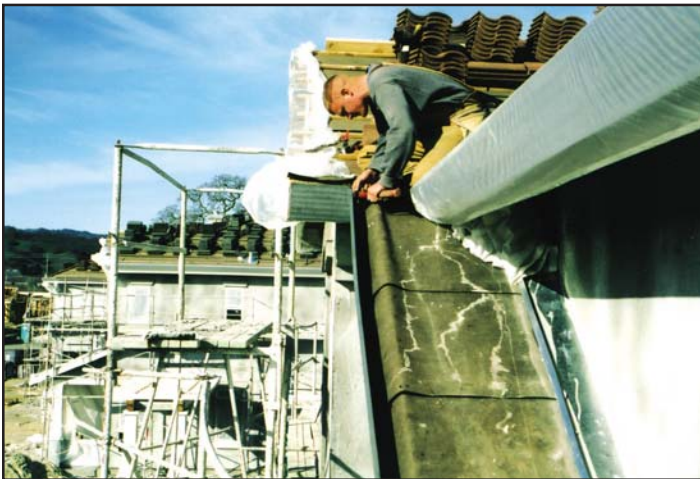
Apprentice Mike Common makes soldering a gutter look easy. Installing residential sheet metal elements and soldering are taught during the second year of the program.
