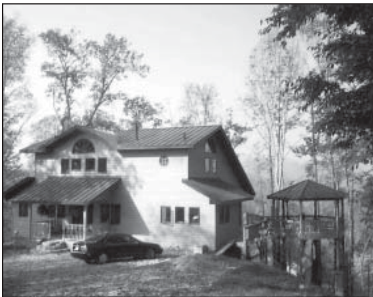
The roof of this private residence was constructed by Morrell Sheet Metal, of Tampa, Fla., and designed by Griffin Design Associates, of Clearwater, Fla., according to specifications in SMACNA's new "Residential Sheet Metal Guidelines."
