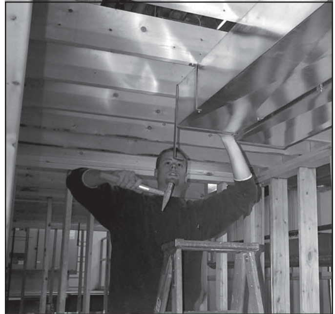
Above: Apprentices learn how to completely install a system from the air conditioner to the gas furnace during their 72-hour residential installation program, which is part of their sheet metal apprentice training. Here, an apprentice is installing a supply duct.
