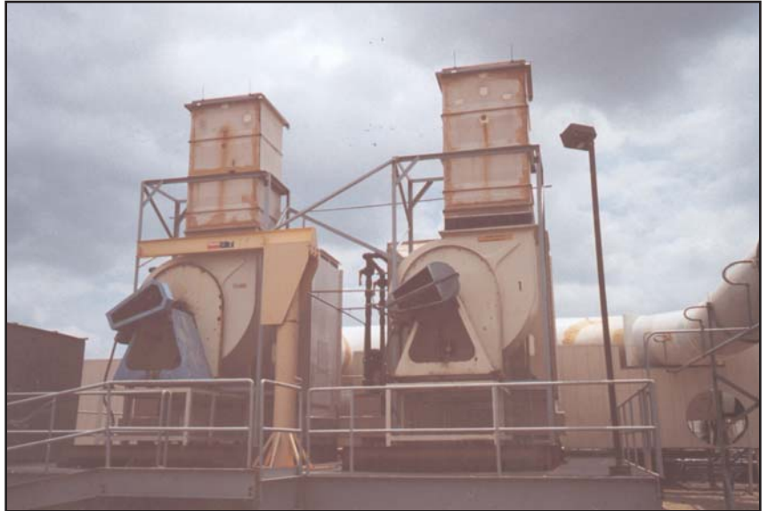
The two scrubbers along with the respective fans, stacks and manifold were installed at National Semiconductor without creating an interference in production.
