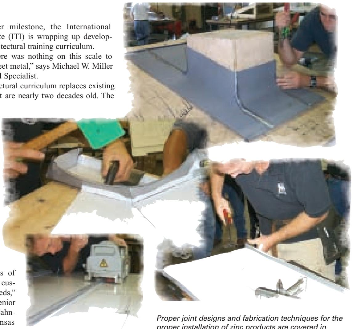
*Proper joint designs and fabrication techniques for the proper installation of zinc products are covered in SMWIA-SMACNA training classes.*
