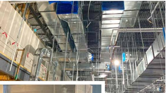
LEFT: The Brandt Companies is currently working on an \$18 million project to fabricate and install all of the ductwork, process piping, HVAC, plumbing and electrical systems at a medical manufacturing facility in Houston.
