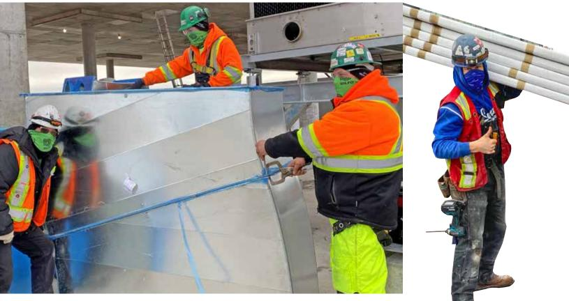
DILFO sheet metal workers install a medium pressure duct main for the office headquarters of a new high-tech company in Ottawa, Ont.
