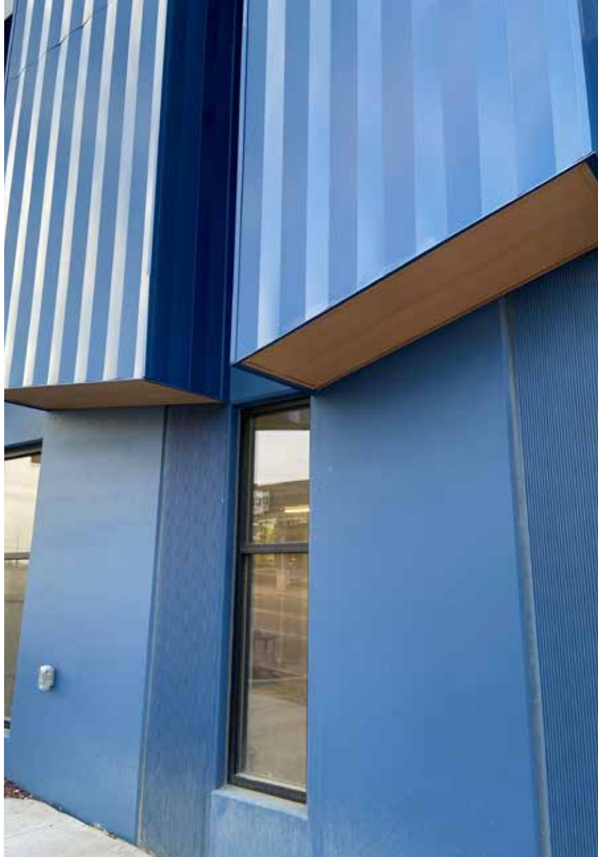
The fabrication of the aluminum dry reveal honeycomb panels began about six months leading up to the start of the jobsite. Photos: Interstate Mechanical Corporation
